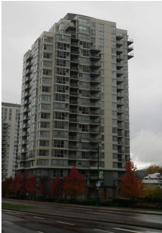
Fig. 2.1.2 Northeast elevation of The Bentley.
